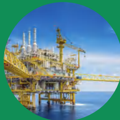
Hydrocarbon processing and petrochemicals
